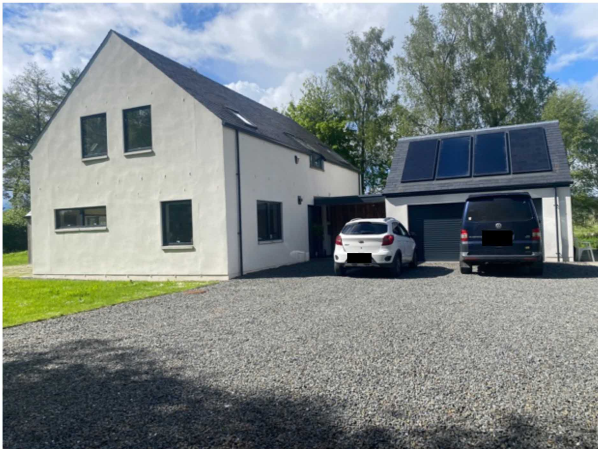
View of Westwater showing the main 1.5 storey house, garage wing, and western wing just visible.
